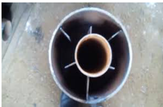
Fig. 9. Water tank and sprayer
