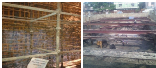
Photographs 1a, b Diaphragm wall of work site
