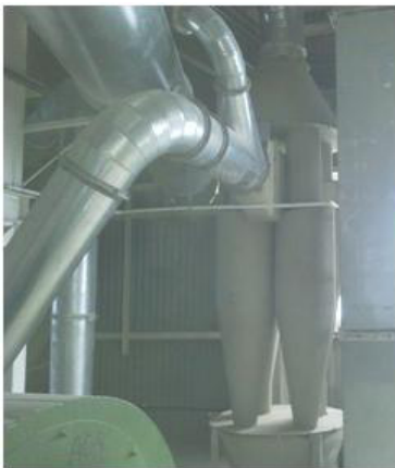
Fig. 1: AS-7 Group cyclone U21-BBC-450 of “Southern Rice Company”, LLC
